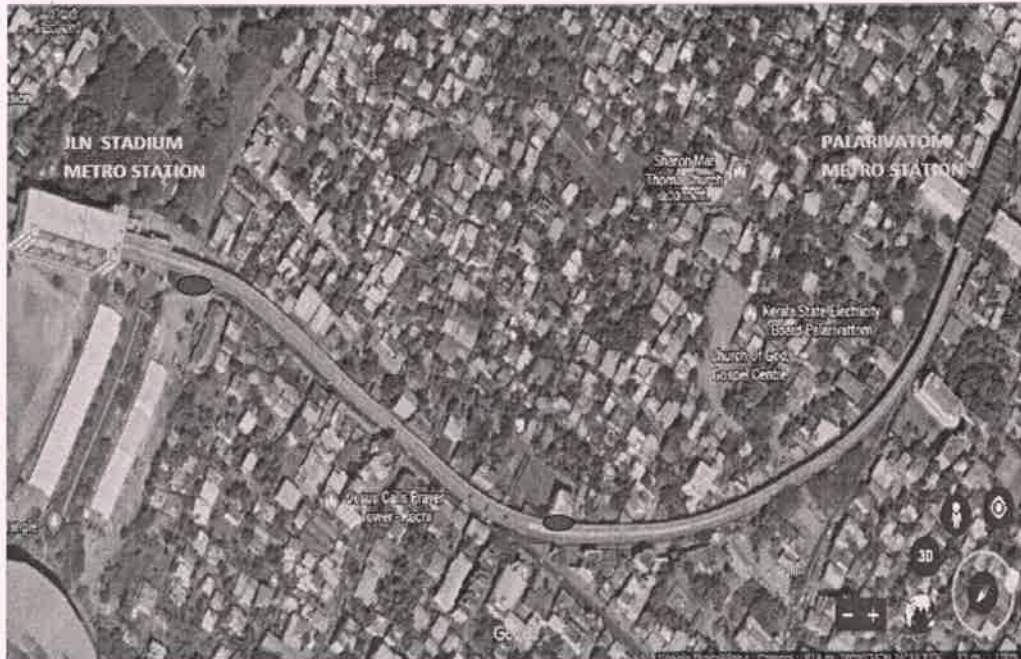
Figure 3.11 Flooding points between Palarivattom and JLN Stadium station
