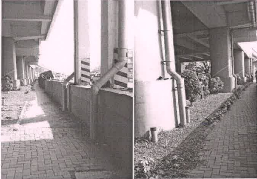
Figure 3.5 Present scenario of rainwater in the metro stations
